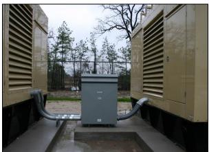
Figure 9: Photo of GenLink DPNL installation
