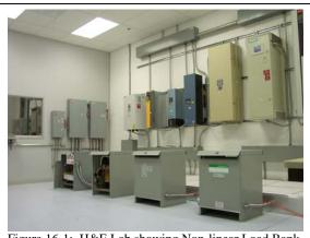
Figure 16-1: H&E Lab showing Non-linear Load Bank
